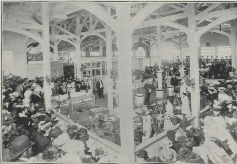
DEMONSTRATION ROOM OF THE NEW DAIRY BUILDING
