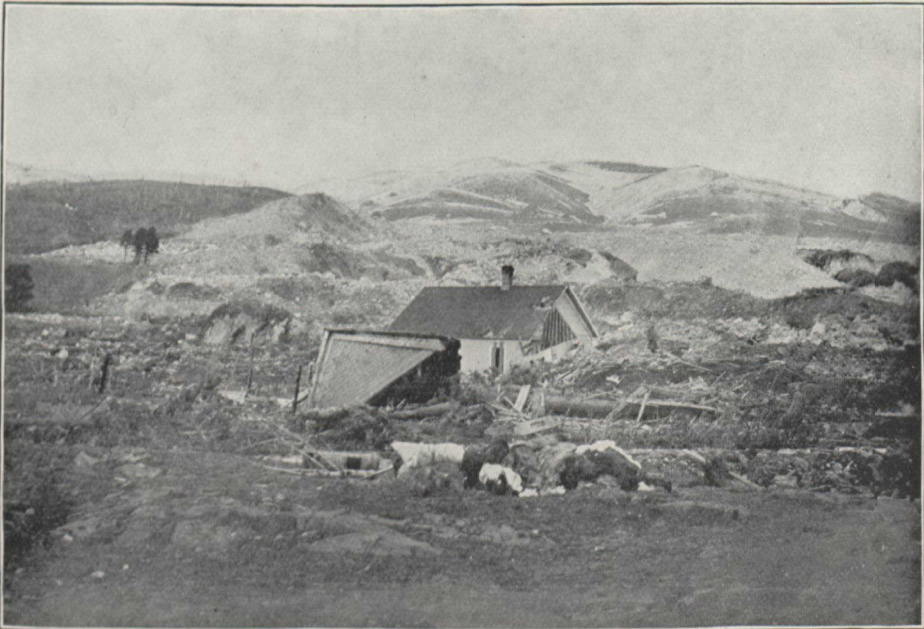
FRANK—SEVERAL HOUSES WERE DESTROYED OR WRECKED AND CARRIED LONG DISTANCES BY THE SLIDE
