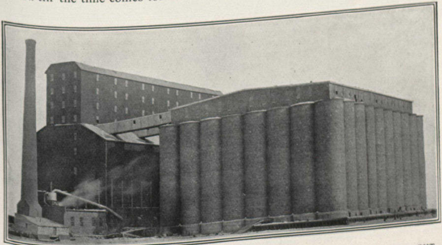
A MODERN TRANS-SHIPING AND STORAGE ELEVATOR—THIS ONE IS AT PORT ARTHUR, ONT., AND IS THE PROPERTY OF THE CANADIAN NORTHERN RAILWAY—CAPACITY TWO MILLION BUSHELS
