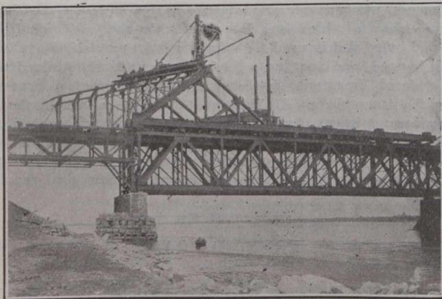
Fig. 2.—Showing Traveller on Falsework, and Camber Blocking.
