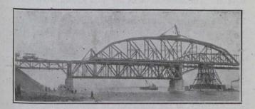
Fig. 3.—Span During Launching, Showing Hauling Apparatus.
