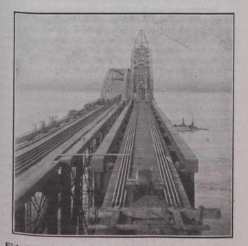
Fig. 4.—End View, Showing Old and New Spans. Also Skidding Track After Launching.
