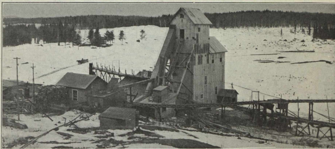
SURFACE PLANT AT NO. 2 VEIN Tough-Oakes mine, Kirkland Lake, Ont.
