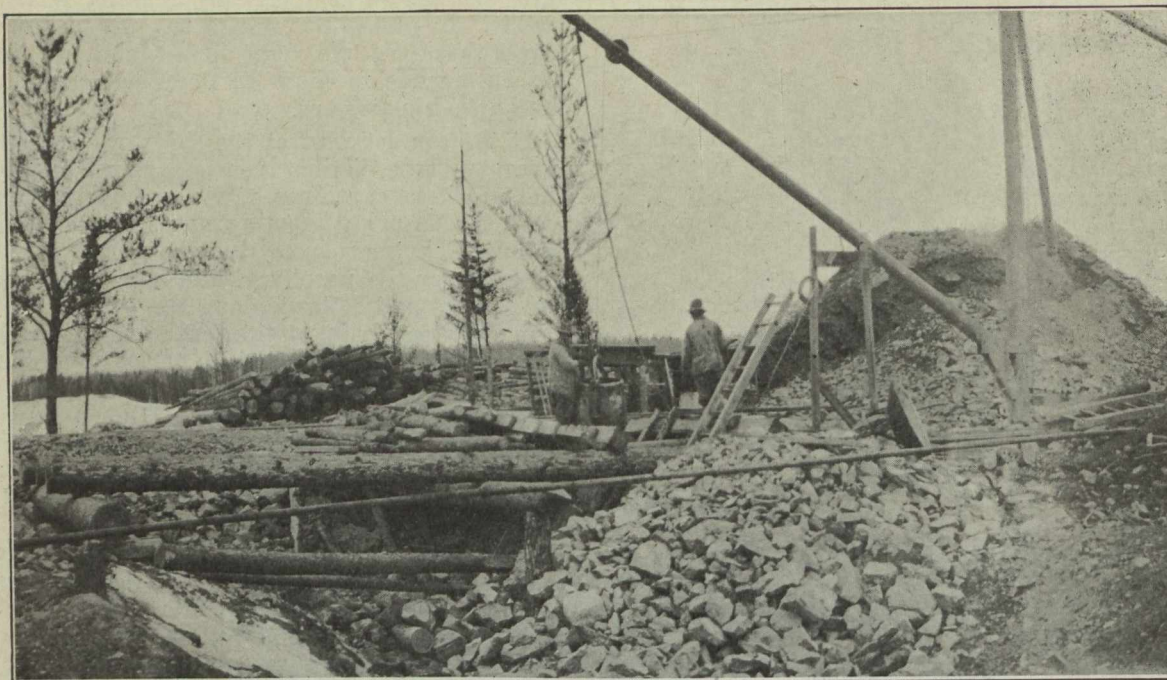
Shaft on No. 3. Vein, Tough-Oakes Mine
