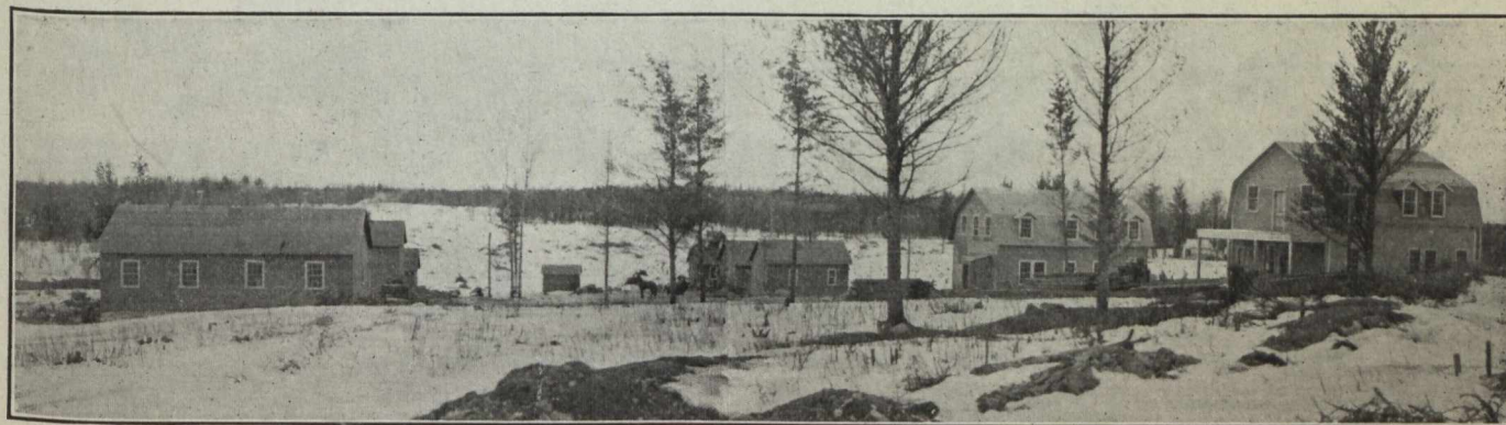
Tough-Oakes Office, Laboratory, Stores and Camp Buildings
