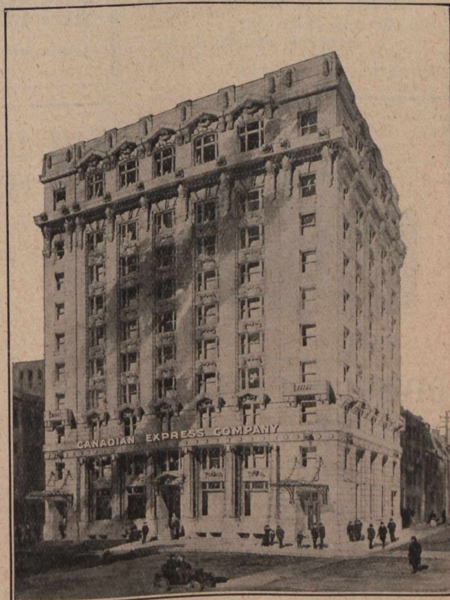
THE CANADIAN EXPRESS COMPANY'S NEW BUILDING, MCGILL STREET, MONTREAL.
