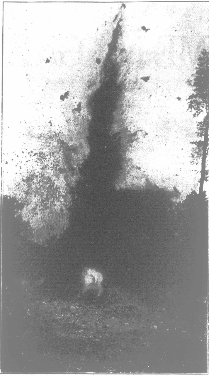
1.—Explosion, 25 sticks 50-per-cent. dynamite, on C. P. R. branch, three miles from Bala, Ont.
