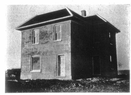
Foundation 30 x 32 feet. Basement walls 7 feet high and 1 foot thick. First storey 9 feet high, walls 10 inches thick. Second storey 8 feet high, walls 8 inches thick.
