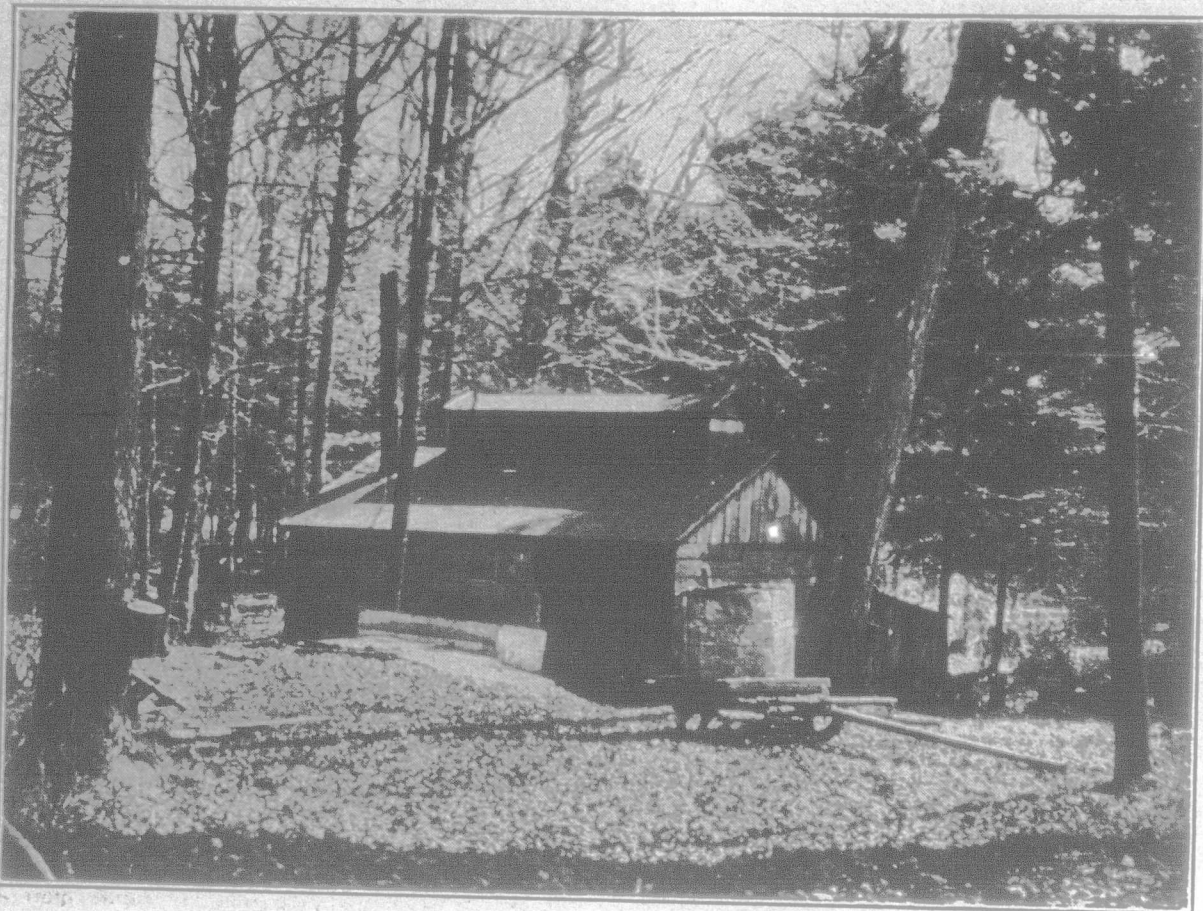
A Modern Boiling House Located in a Maple Bush.
