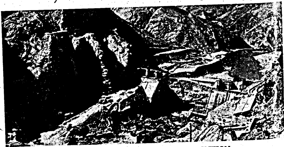
THE WARSAK DAM UNDER CONSTRUCTION
