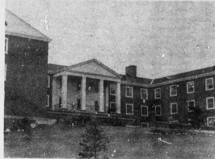
Lady Dunn Hall, Tibbits Hall and the Health Centre are in the rear.
