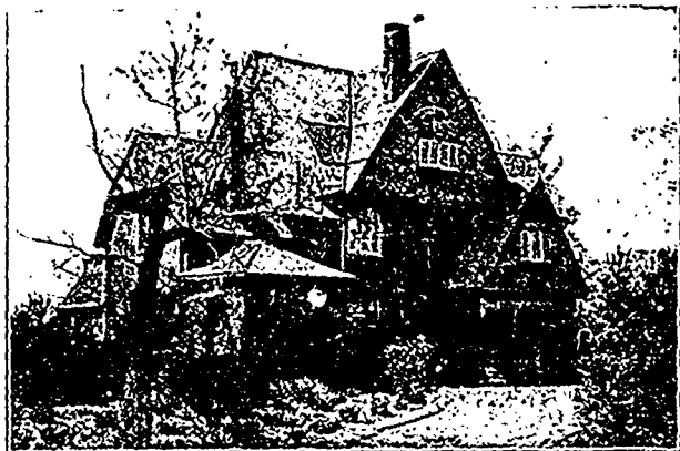
If you are thinking of building a home, call on, or write. Phone M. 1372. R. J. EDWARDS, Architect, 18 Toronto St., TORONTO
