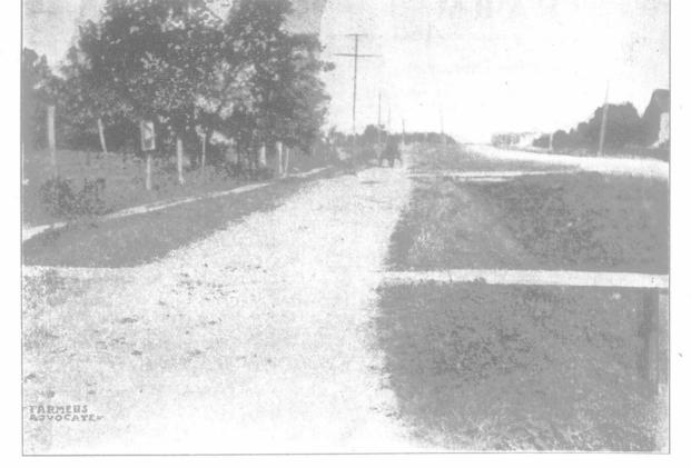
CLAY DRIVE ON ROAD SIDE IN KILDONAN ON WHICH TEAMS GO IN DRY WEATHER AND WHEN THE CITY IS APPROACHED RIGS BUMP OVER CROSSINGS AND INTO HOLES.
