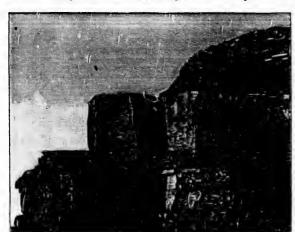
Fig. 10. Front of limestone quarry at edge of escarpment, Hamilton, showing disintegration of rock by weathering; rock almost wholly disintegrated at top.
