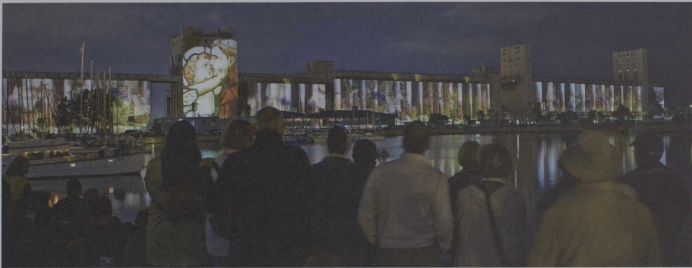
The largest multimedia outdoor architectural projection in the world: the grain silo operated by Bunge North America (see page 28) in the Port of Québec becomes a 600 m x 30 m screen for the summer production of Le Moulin à images (The Image Mill).
