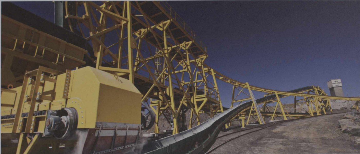
Vale's New Demonstration Plant Featuring Canadian Innovative Hauling System Technology. Photo courtesy of Rail-Veyor Technologies Global Inc.
