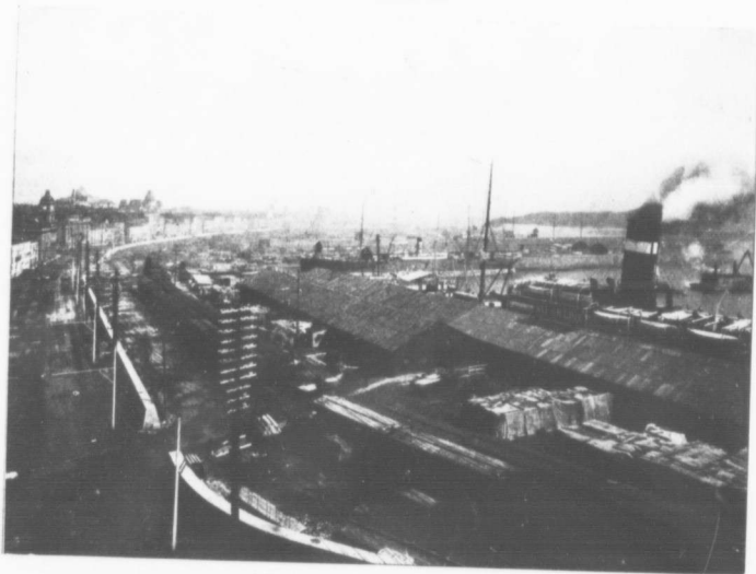
A PORTION OF MONTREAL HARBOR.
