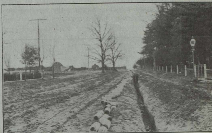
Tile Drains More Desirable than Blind Drains.
