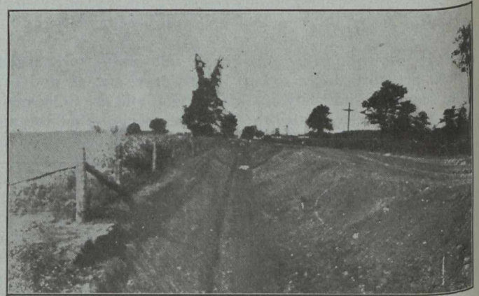
Ditches Such as This are a Menace.
