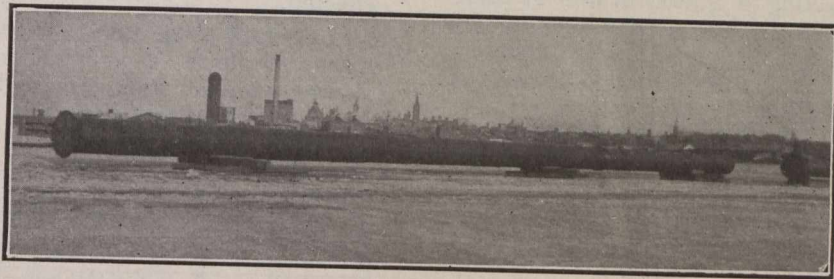
Fig. 1.—A Length of Pipe Ready for Relaying
