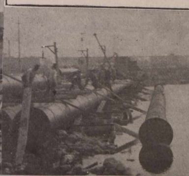
Fig. 3. Launching 200 Ft. of Pipe.
