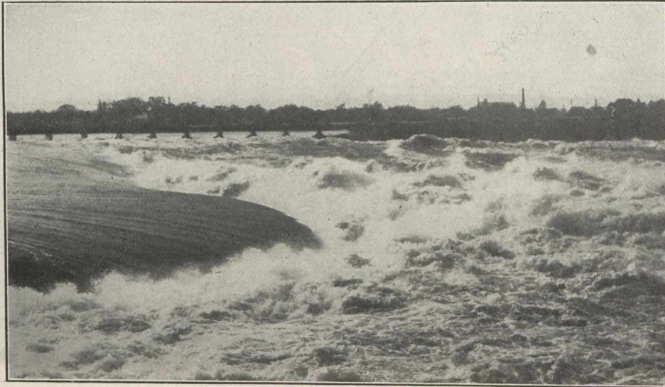
Dam in Spring Flood, May, 1909.
