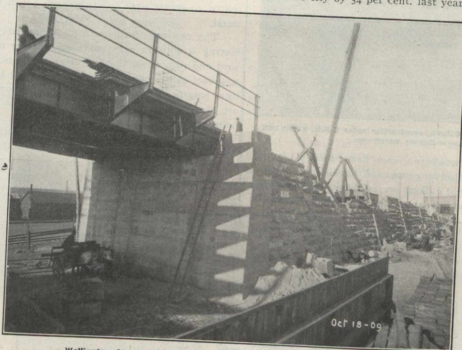
Wellington Street Viaduct, Ottawa, Concrete Abutments and Masonry Retaining Wall.
