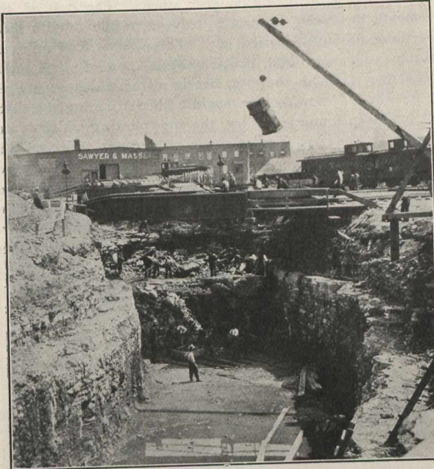
Waterworks Aqueduct, Ottawa, construction under C.P.R. tracks and Sawyer-Massey warehouse.
