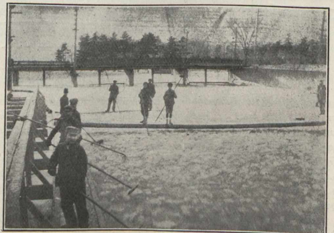
Forebay at Hull Electric Power House. Forebay full of Slush, Frazil Ice, etc.
