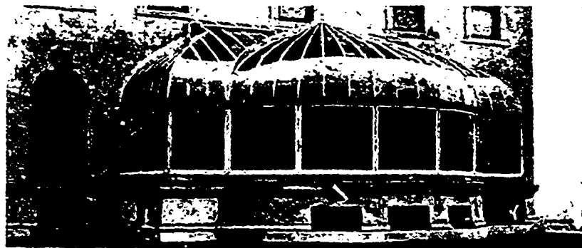
ERECTED FOR M. E. DAVIS, MONTREAL, CANADA.
