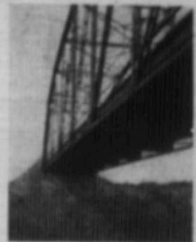
A 150-ft. Steel Span on Re-inforced Concrete Abutments
