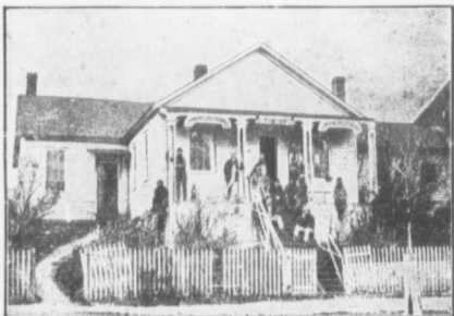
FIRST GOVERNMENT OFFICES ON MAINLAND OF BRITISH COLUMBIA, AT NEW WESTMINSTER.
