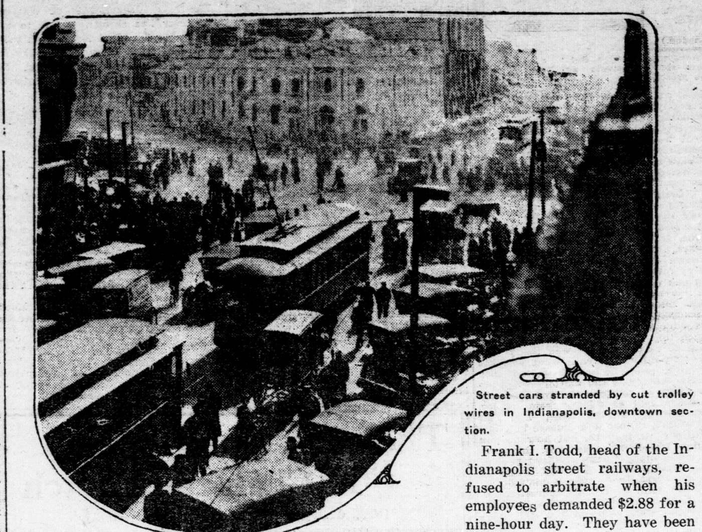
Street cars stranded by cut trolley wires in Indianapolis, downtown section.
