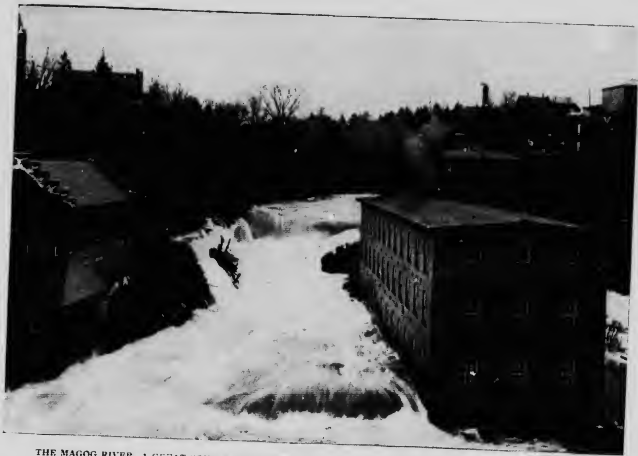
THE MAGOG RIVER—A GREAT SOURCE OF POWER. THE COMPANY'S WATER POWER BEFORE DEVELOPMENT
