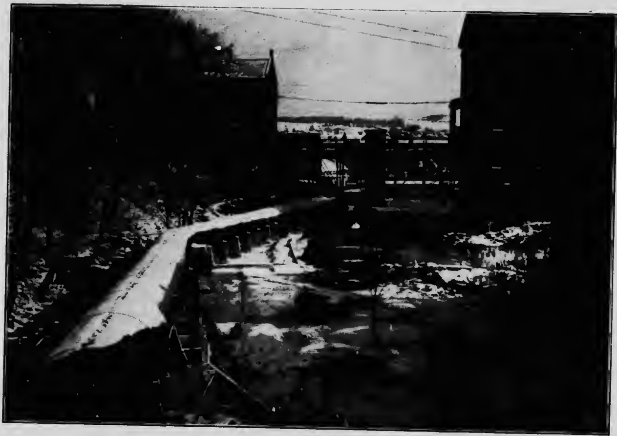
THE PENSTOCK OF THE COMPANY, 9 FT. 6 IN. IN DIAMETER AND 650 FT. LONG, CARRIED ON CONCRETE COLUMNS 16 FT. APART
