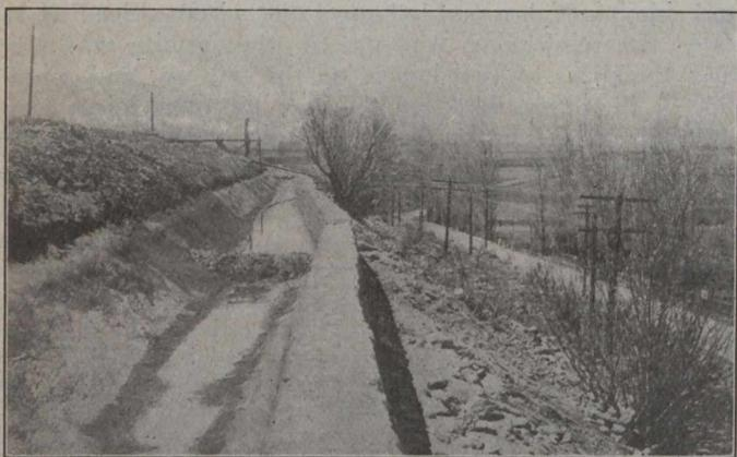
Fig. 6.—Showing Finished Canal Ready for Filling
