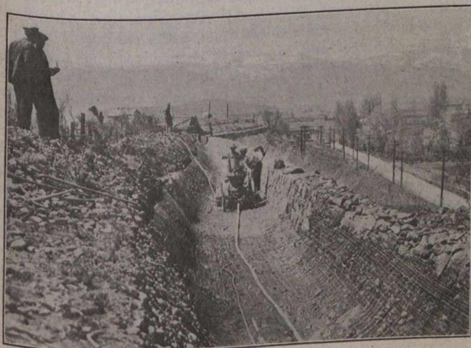
Fig. 2.—Reinforcing in Place Ready for Gunite
