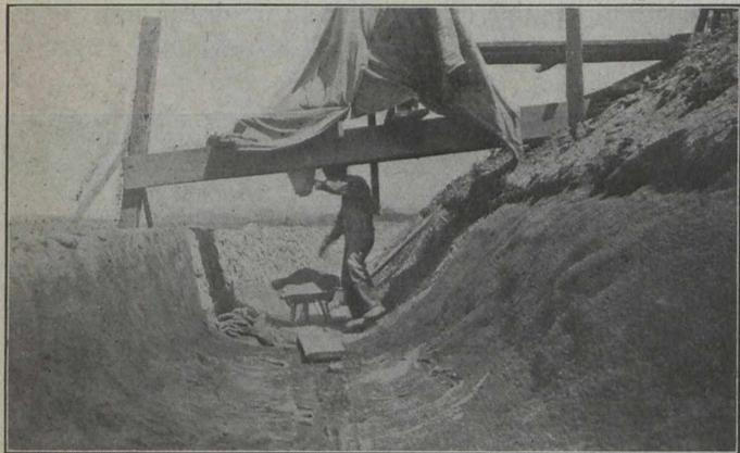
Fig. 5.—Loading Wheelbarrow from Hoppers
