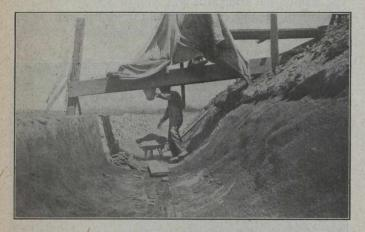
Fig. 5.—Loading Wheelbarrow from Hoppers
