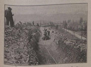
Fig. 2.-Reinforcing in Place Ready for Gunite
