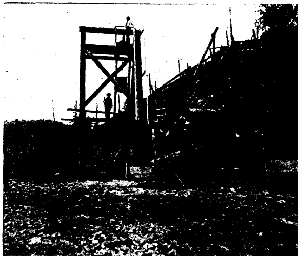
Gallows Frame and Hoist in Position.
