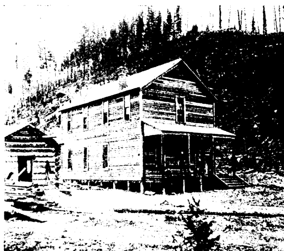
Men's House—Nearing Completion.
