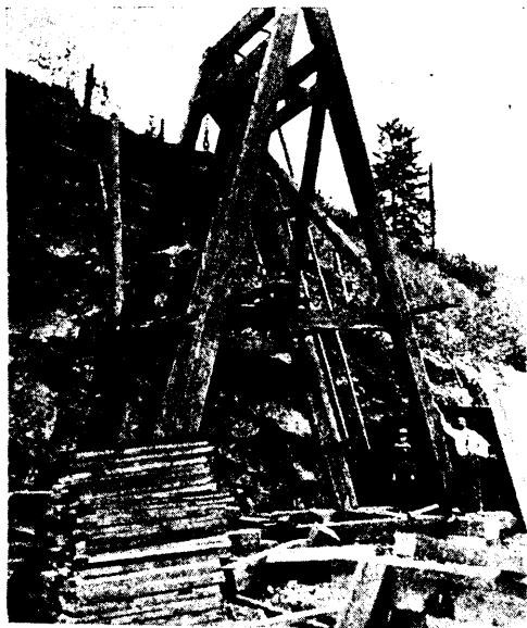
Building Gallows Frame.
