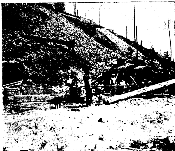
Commencing Erection of Plant.
