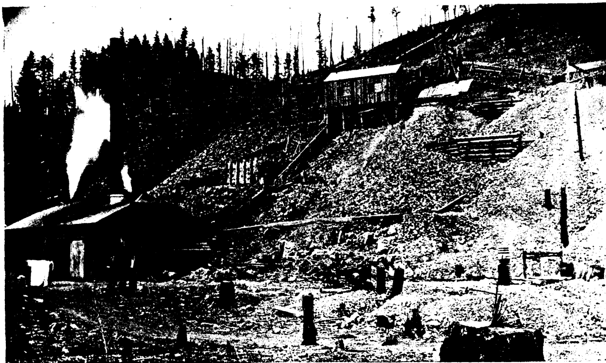
General View of Works.
