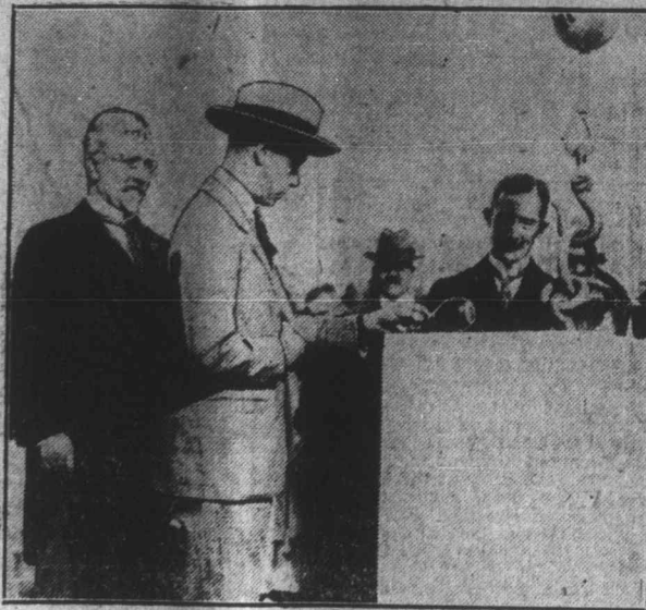
By reason of too much handshaking during his visit to Cape Town, the Prince of Wales contracted a swollen wrist. The Prince is shown laying the Foundation Stone of the New Cape Town University with Sir J. C. Beattie, Principal, just behind. Note the Prince laying the stone with his left hand as his right hand is bandaged.
