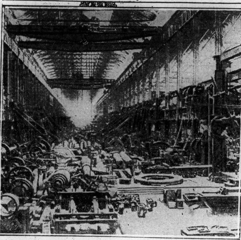
MACHINE SHOP NO. 4 AND CRANES WHICH SAVED GUNS. While the flames were at their height in the great fire which destroyed the big machine shop of the Bethlehem Steel Company, at South Bethlehem, Pa., the electric travelling cranes on the main floor were operated to remove as many of the eight hundred guns in the building as possible. Two hundred finished guns for the Allies were saved in this manner, as well as much unfinished artillery. Nearly one thousand machines, however, together with the tools of the workmen, are a total loss. The fire caused a loss of $2,000,000, and greatly delays deliveries to the Allies.
