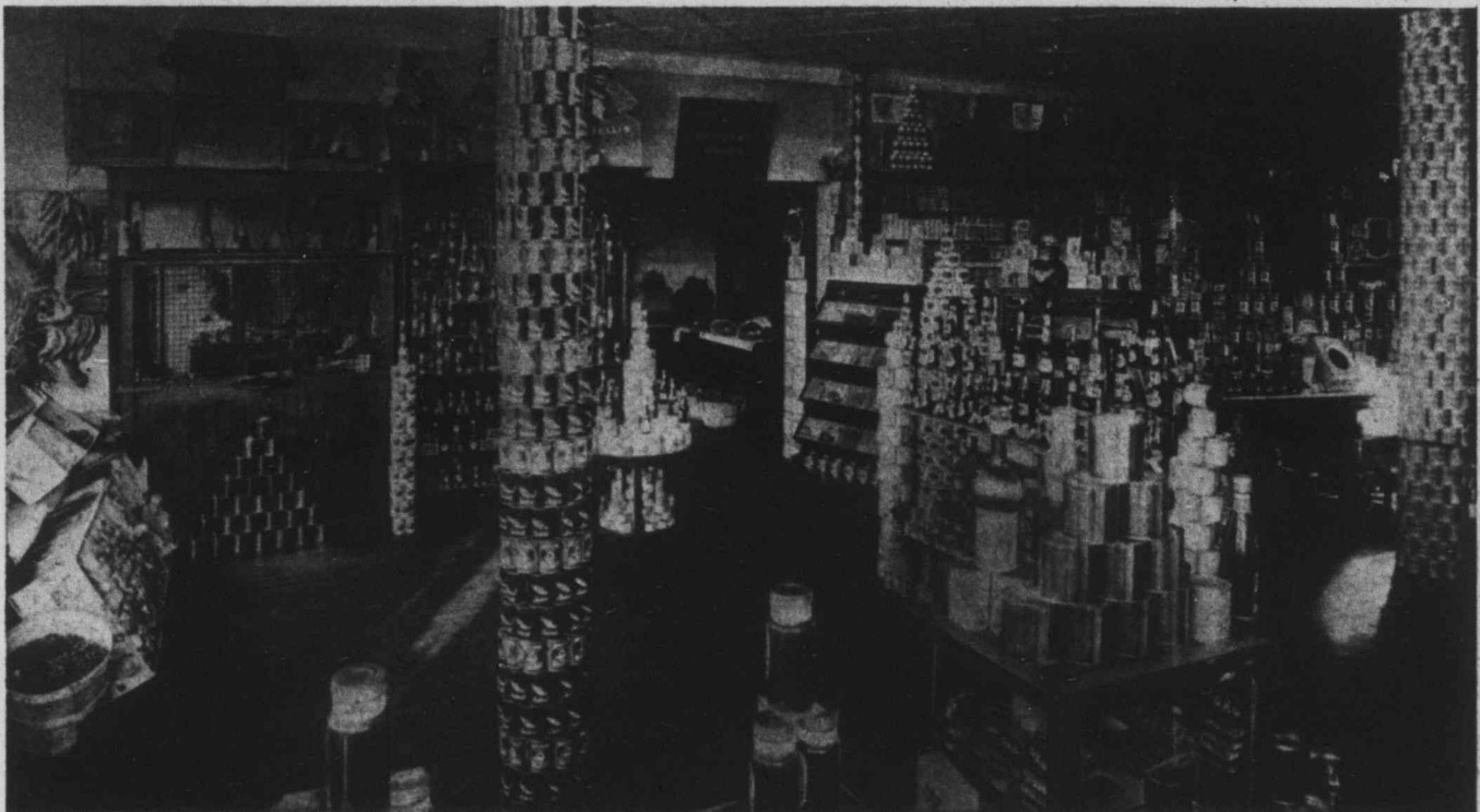
The interior of the L. Krivel Grocery and Meat Store, Corydon Avenue, Winnipeg, showing the meat department in the distance, with a glimpse of the office that serves both departments.
