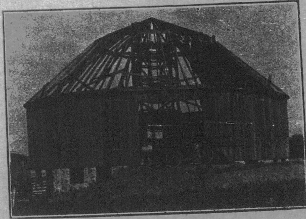
A Round Barn in Course of Construction.
