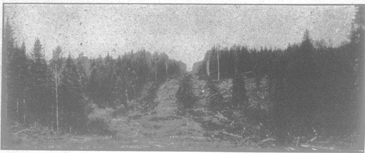
New Government Road Being Cut Through near Cochrane, Ont.
