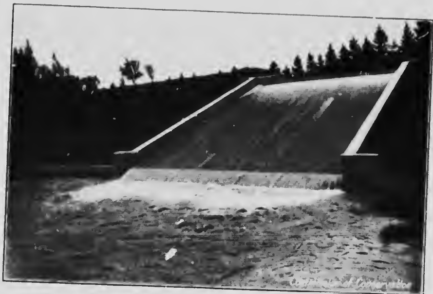
St. Catharines Water-works - Spillway for Surplus Water
