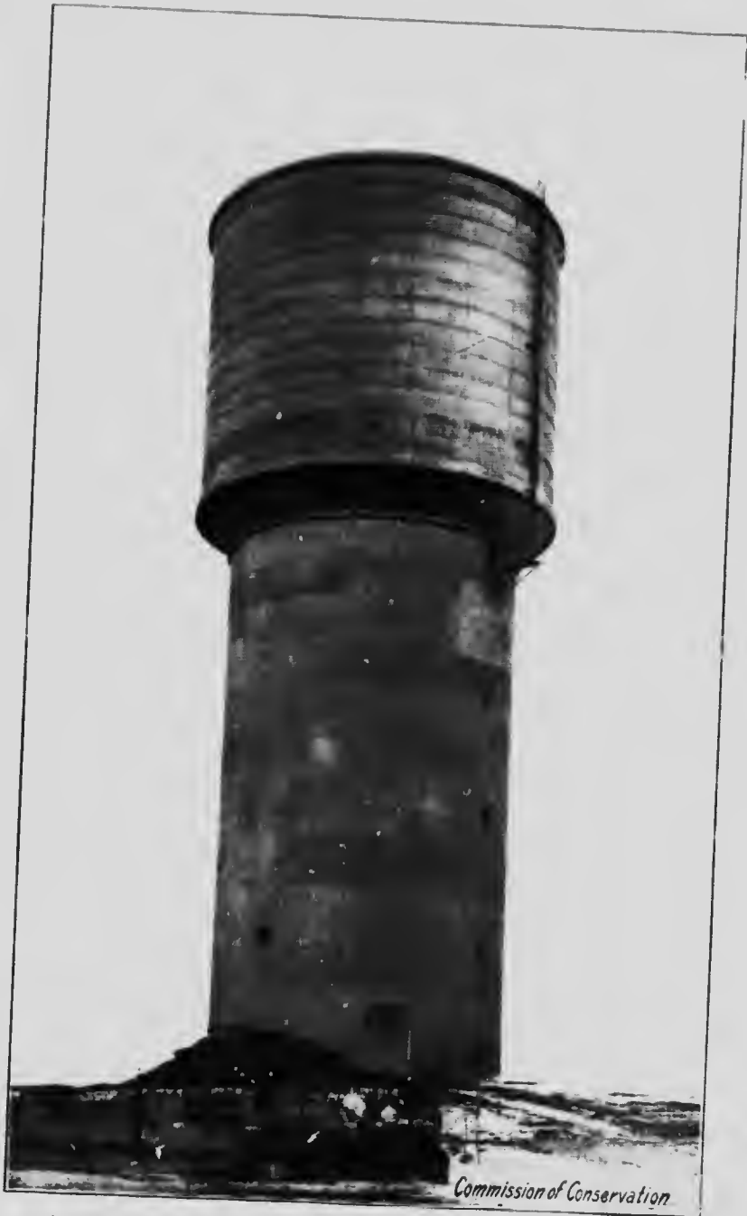
Berlin Water-works—500,000 gal. Concrete Elevated Water-tower
