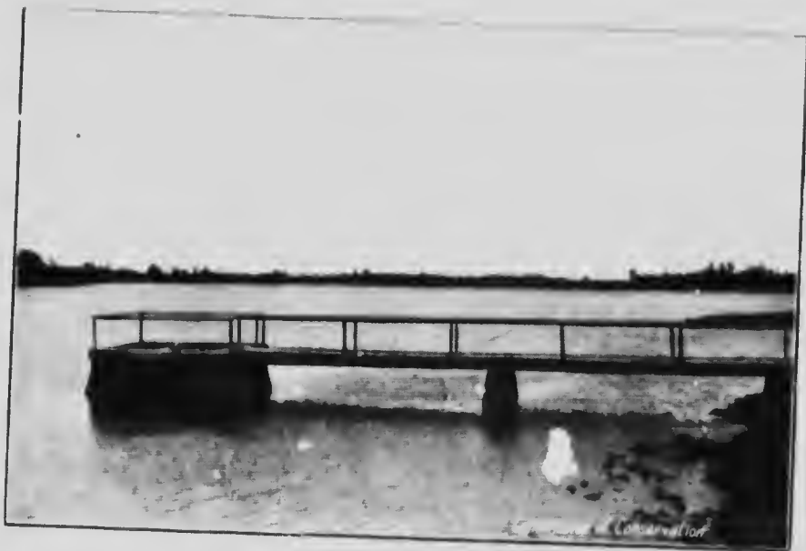
St. Catharines Water works - 24 in. Intake
