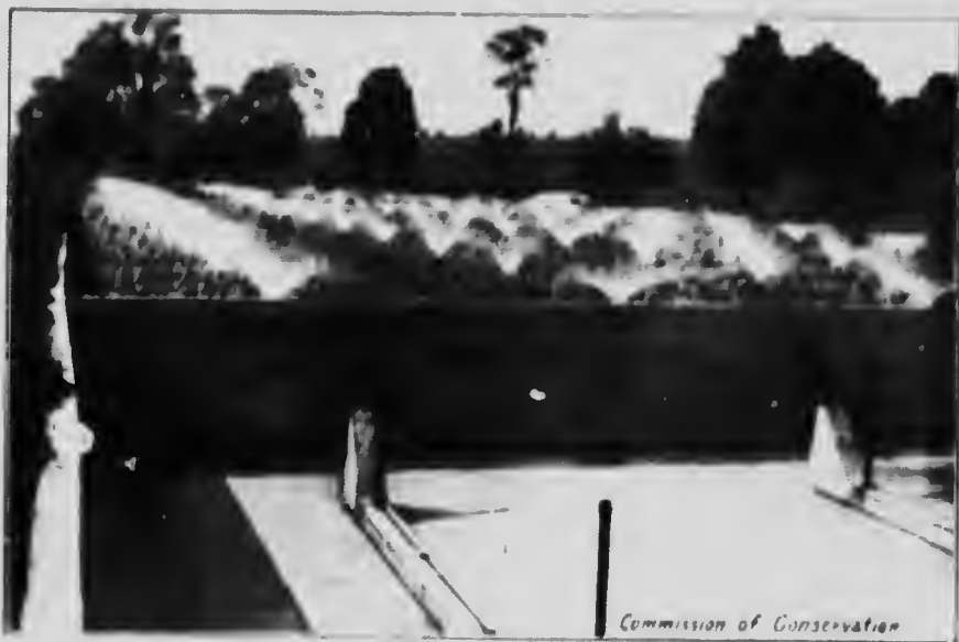
Stratford Sewage Disposal Works - Sprinkling Filters - Summer View
