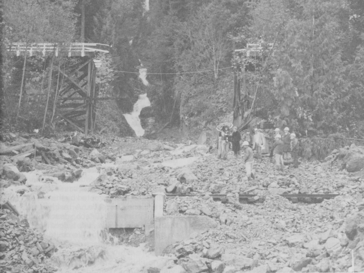
Local residents and construction crew gaze at the chaos created in the wake of the "M" Creek mud slide, which demolished the middle section of the highway bridge. Nine people were killed in the disaster.
