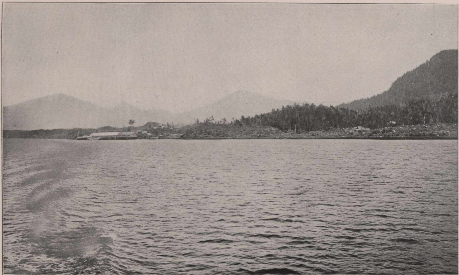
GENERAL VIEW OF WHARF AND TOWNSITE—PRINCE RUPERT.
