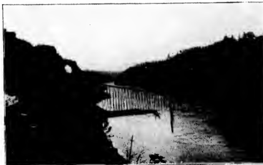
Wreck of the Old Suspension Bridge.
