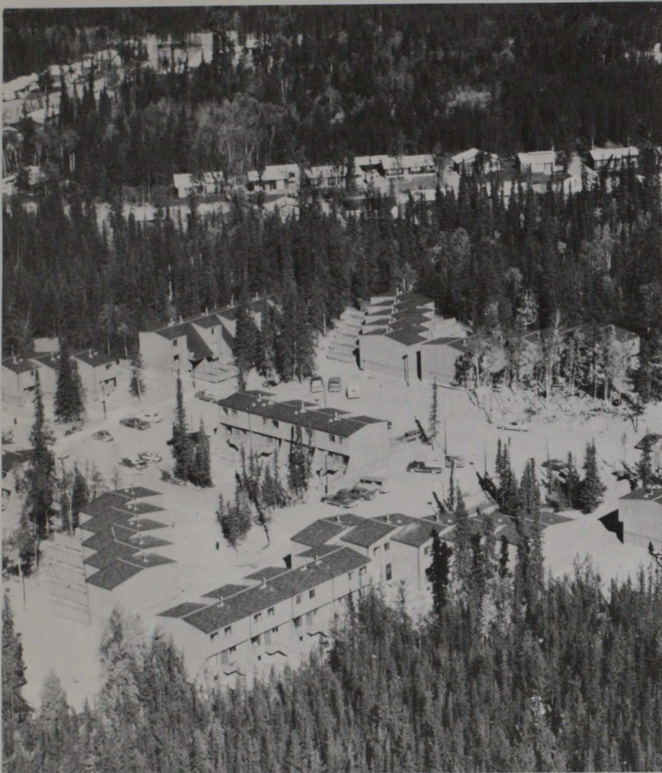
Leaf Rapids, Manitoba is a new mining town, designed to overcome the social and economic problems which can make life unpleasant in resource-based settlements.
