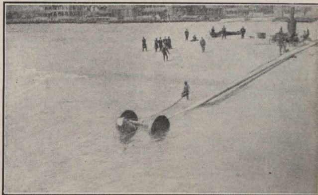
Fig. 1.—Twelve-Inch Pipe, 1,000 ft. Long, Being Submerged After Assembling on Shores.
