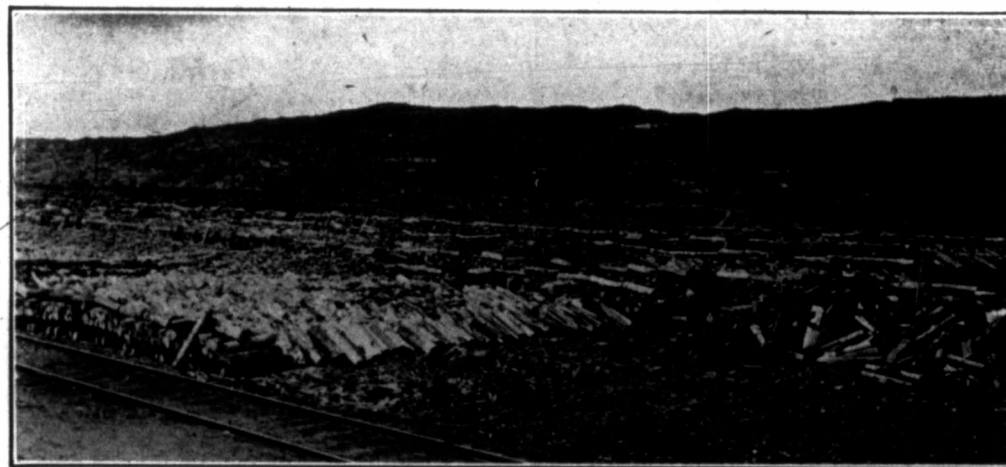
Roasting nickel-copper ore
