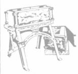
**DUNN Hollow Concrete Block Machines** are in use from coast to coast, and every one giving the best of satisfaction. Concrete blocks make the handsomest, most durable and cheapest building material. They are simply and quickly made on the DUNN MACHINE; and the
