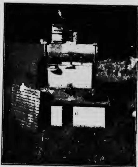
FIG. 3.—Sibbald hot-water Wax Extractor.
