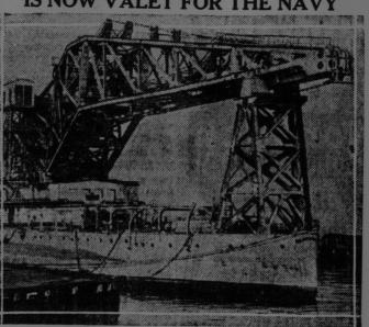
Whenever a battleship at sea needs its uniform adjusted, such as a new turret or a new gun lifted into place, the crane ship Kearsarge is called for. The crane has lifting capacity of 250 tons. Yes, it's the same Kearsage that used to be the proud battler.
