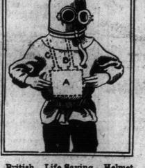
(A) Oxylithe Container, an Oxygen Generator, Permitting Air to Be Used Again and Again. (B) Inhaling Tube.
