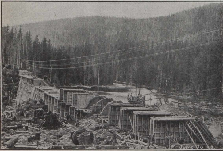
Fig. 1.—General View of the Jordan River Dam During Construction.
