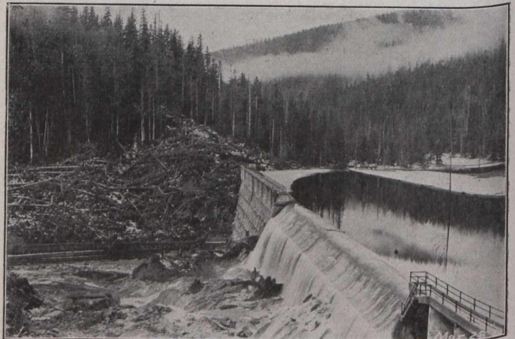
Fig. 3.—Jordan River Dam Completed.
