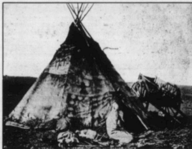
Along the Old Trail
