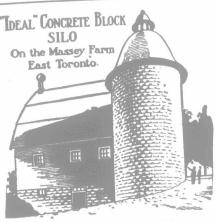
**Erected at Dentonia Park Farm** for Mrs. E. D. Massey. 34 feet high-15 feet diameter-capacity 180 tons. Built of "Ideal" Blocks.
