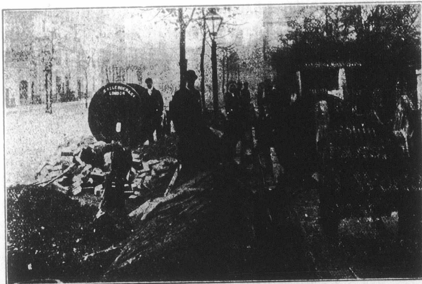
Laying Callender Mains at DONCASTER.
