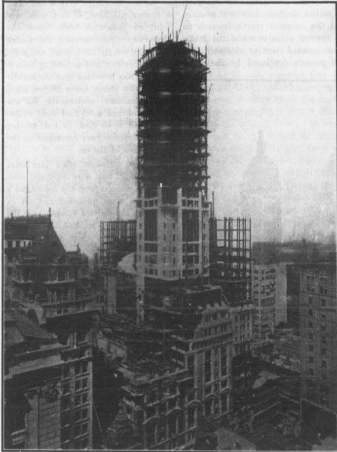
VIEW OF SINGER BUILDING TOWER DURING ERECTION.
