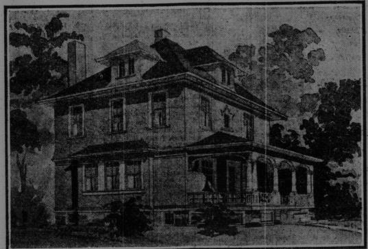
This design represents a house 30 feet front by 28 feet deep, exclusive of the piazza. The latter extends the full width of the front and is 9 feet wide. The external appearance of this house is symmetrical, with the wide projected eaves and timber brackets on the under side, the treatment of of the piazza and main roof being the same. The cornice members of the piazza are carried around the house and the upper portion of the walls are shingled, while the first story is cov-
