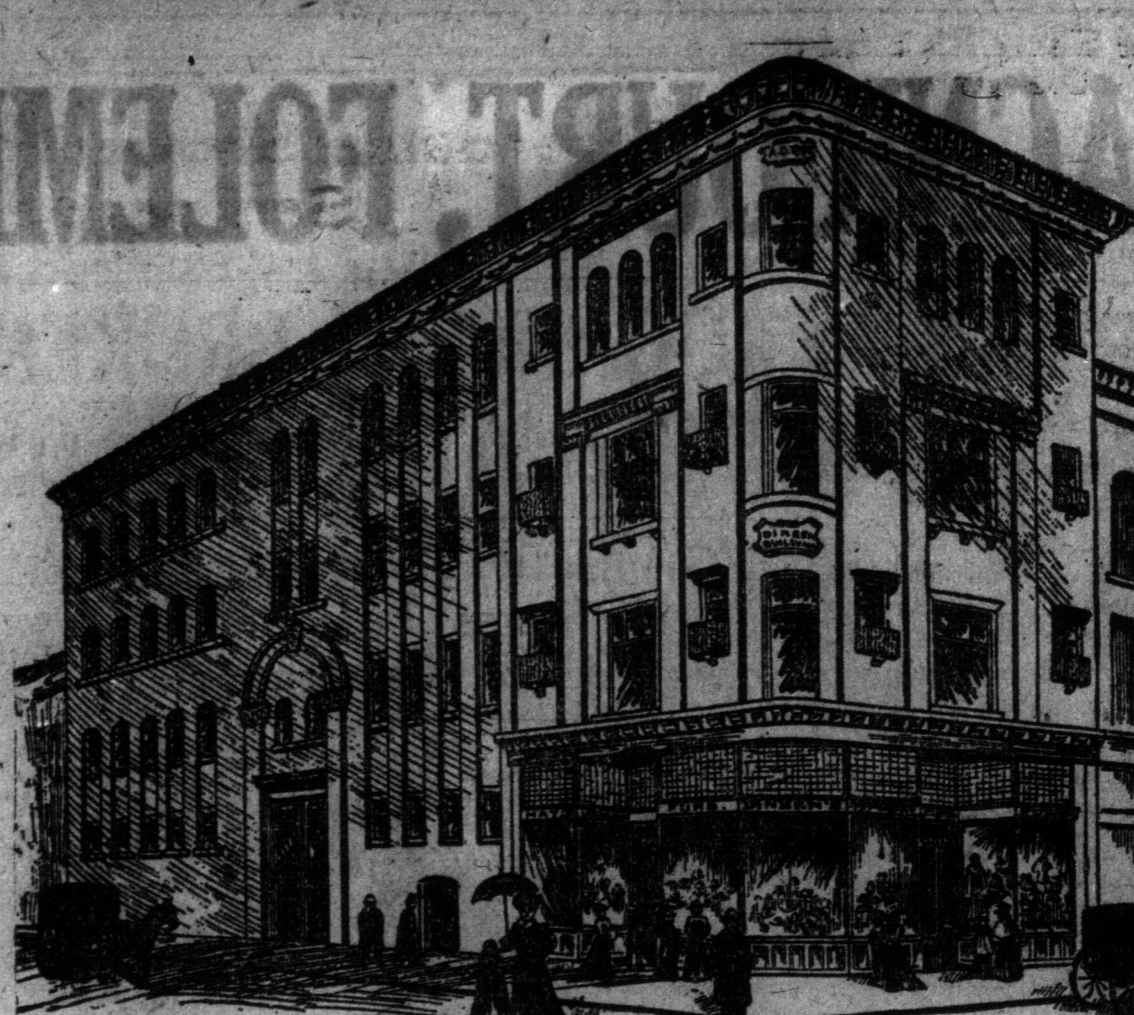
This is the Fine Building that was Guted by Fire.
