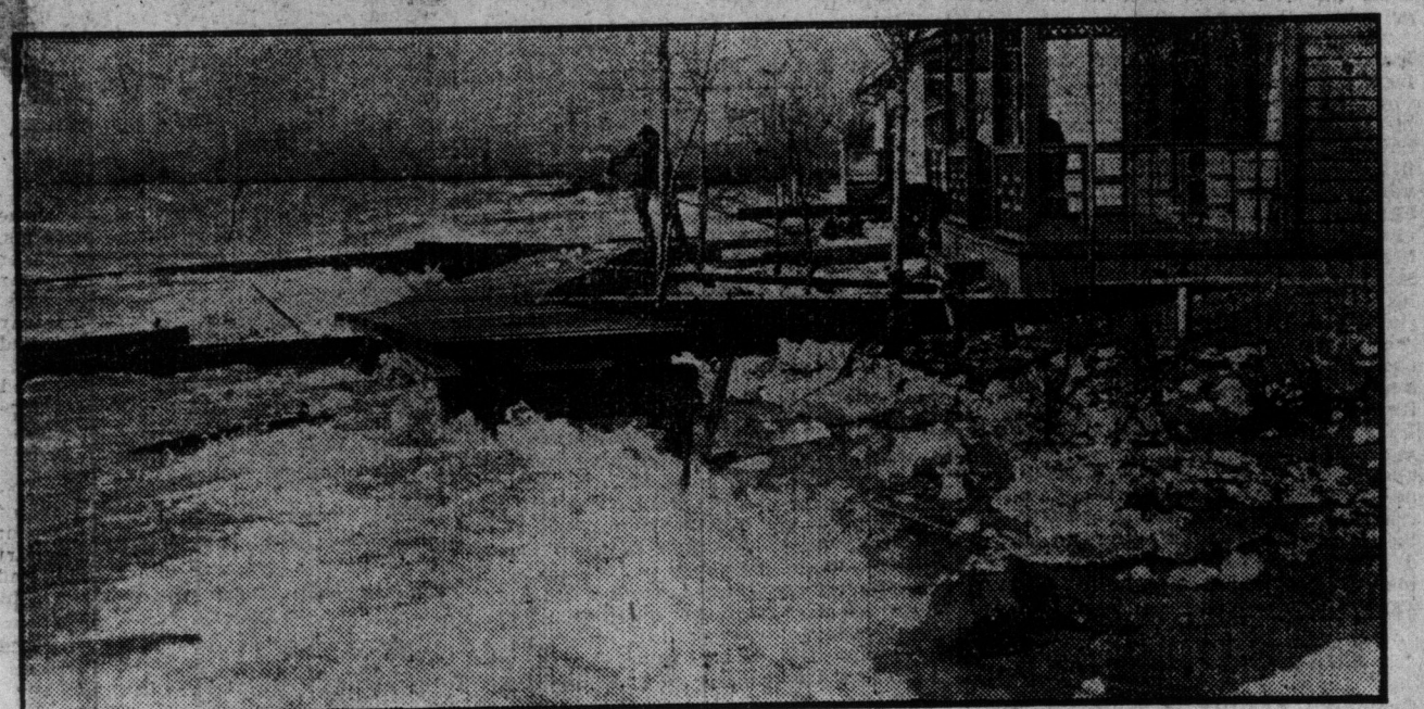
THE RECENT DAMAGE BY WIND AND WAVE: What it Looks Like on the Western Sandbar.
