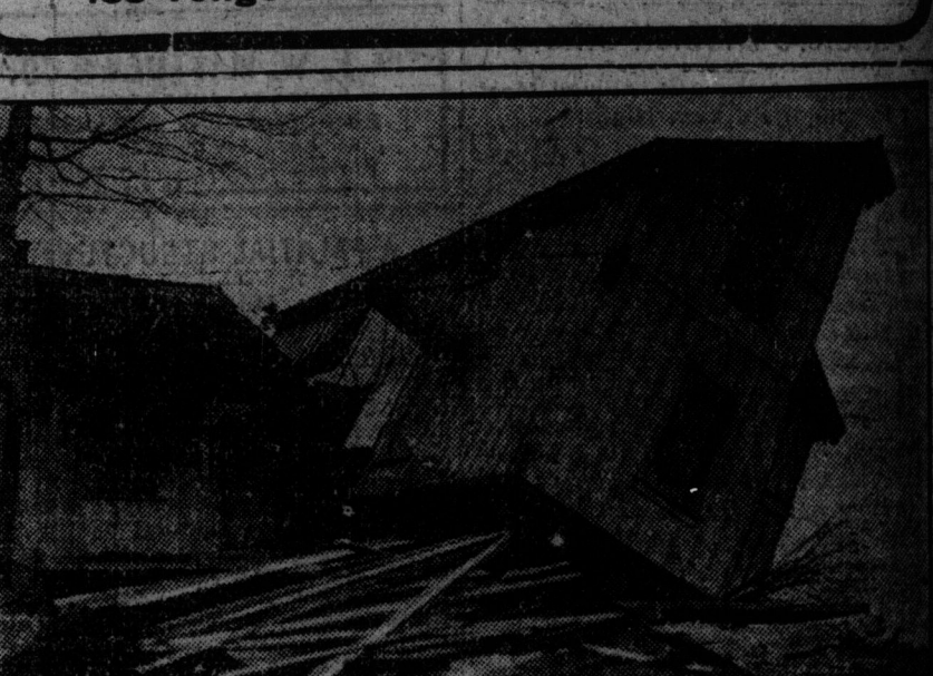
THE RECENT DAMAGE BY WIND AND WAVE: How Underrated at Kew Beach.
